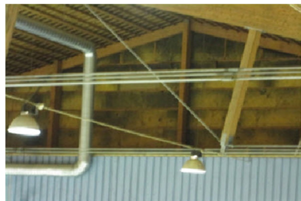
Fig. 2. Mould growth on the ice rink structure.
