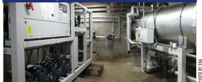
PHOTO 1 The CO 2 pack providing 250 kW (71 tons) cooling capacity and the 2.5 m 3 (88.3 ft 3 ) CO 2 receiver.
